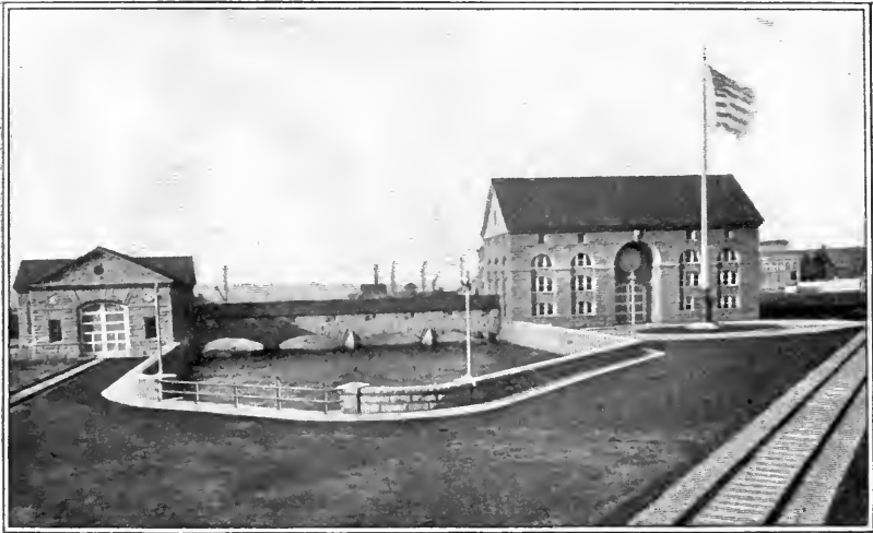
The Exterior of the Power House at Niagara Falls
